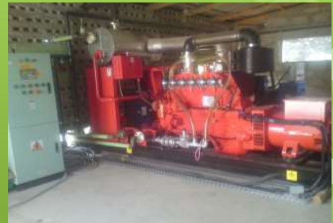
DIESEL GENERATOR OF HPW (150 KVA) WHICH RUNS ON THE GENERATED BIOGAS (ADEISO, E/R)
